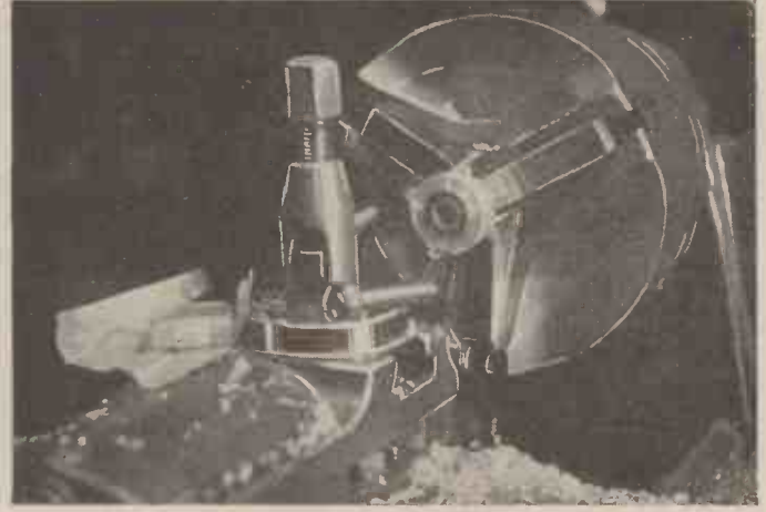
Fig. 10.—The finished main bearing housing bored and turned at one end. Note the ball race fitted with a temporary handle, lying against the tool post, for use as a plug gauge.
