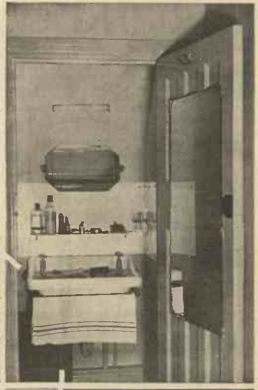
A built-in cupboard for the lavatory basin. The tubular lamp is automatically illuminated as the door is opened. Note the mirror on the inside of the door.
