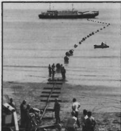
Preliminary submarine cable laying activity. Reproduced by kind permission of British Telecom.
