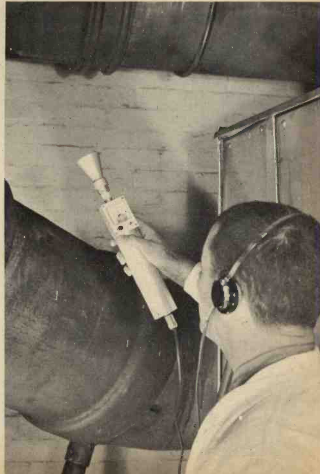
The location of a leak is now nearing completion with the Ultrasonic Leak Detector
