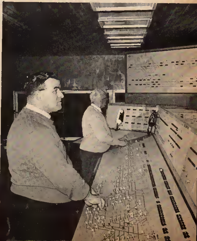
Part of the control panel in Rugby signal box, from which remote interlockings are operated by an electronic supervisory system
