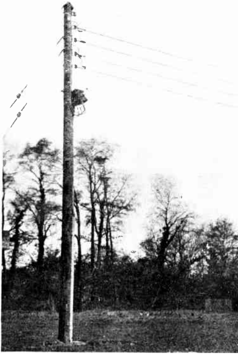
Fig. 12.—TERMINAL POLE FOR LOW TENSION DISTRIBUTION.
