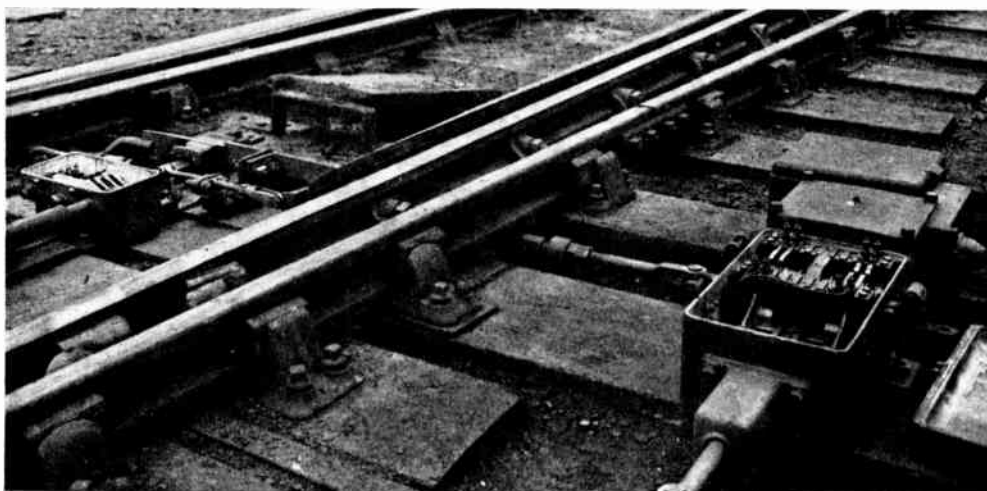
Fig. 4. —THE POINT MACHINE AND DETECTOR MECHANISM.
