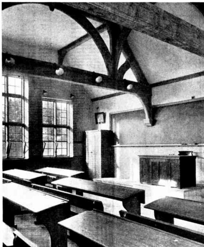
Fig. 4.—CLASS ROOM LIT BY SIDE REFLECTORS WITH EXTRA ROW ON BEAM ACROSS THE ROOM.
