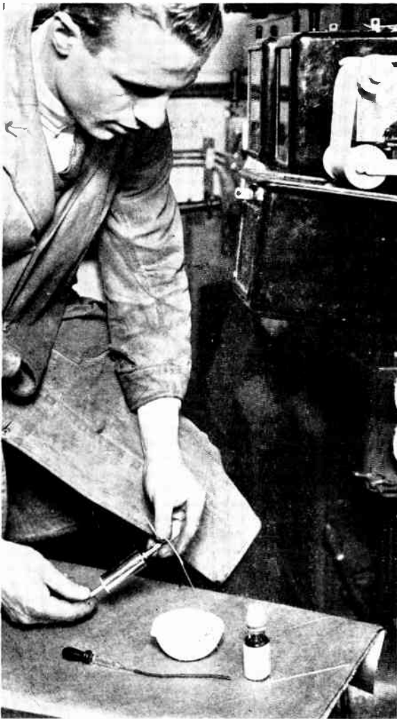
Fig. 21.—CLEANING OUT THE TUBULAR PEN WITH GLYCERINE, AFTER LONG SERVICE.
