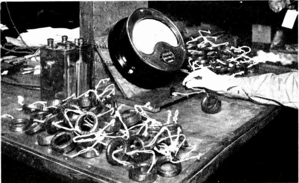
Fig. 17.—MEASURING THE RESISTANCE OF COILS AS A WORKSHOP ROUTINE TEST.
