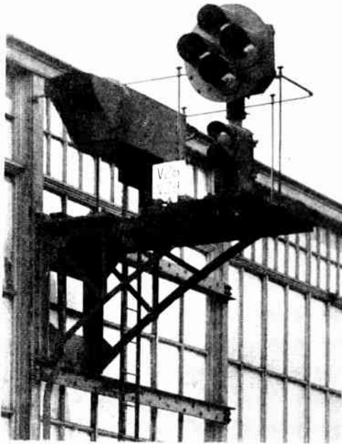
Fig. 2. WESTINGHOUSE FOUR-ASPECT (CLUSTER TYPE) AND TWO-ASPECT (VERTICAL TYPE) COLOUR-LIGHT SIGNALS AND OPTICAL ROUTE INDICATOR (ON LEFT).
