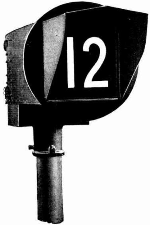
Fig. 3.—WESTINGHOUSE OPTICAL ROUTE INDICATOR. FIGURES 11 INCHES HIGH.
