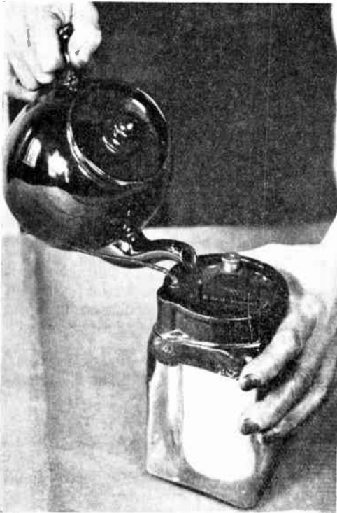
Fig. 4. —THE CORRECT METHOD OF FILLING A JAR WITH SAL-AMMONIAC SOLUTION.
