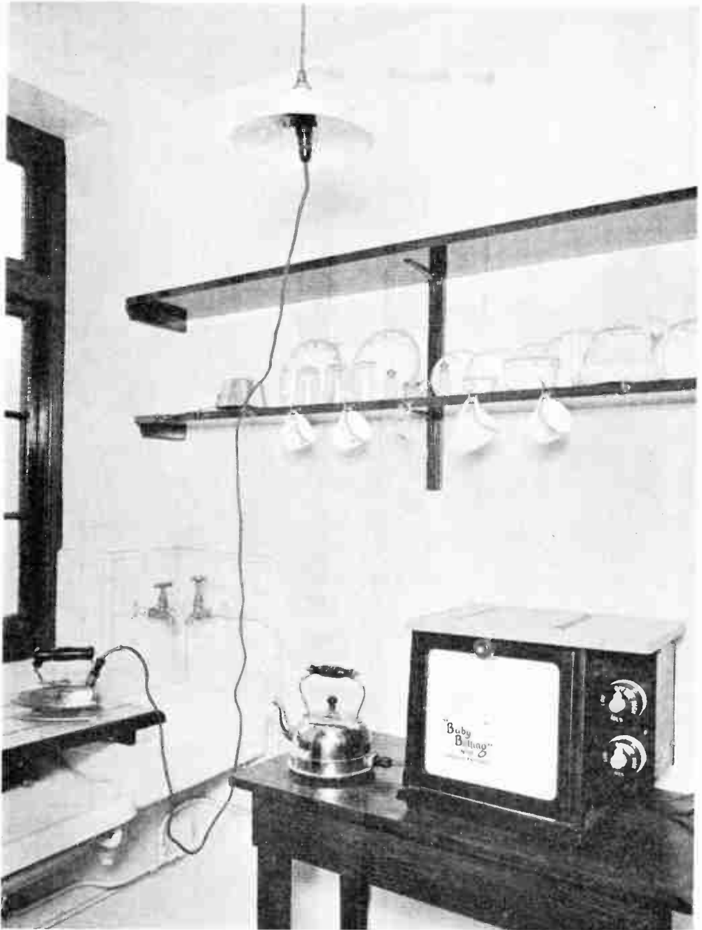
Fig. 3.—THREE USES OF ELECTRICITY IN THE KITCHEN.
