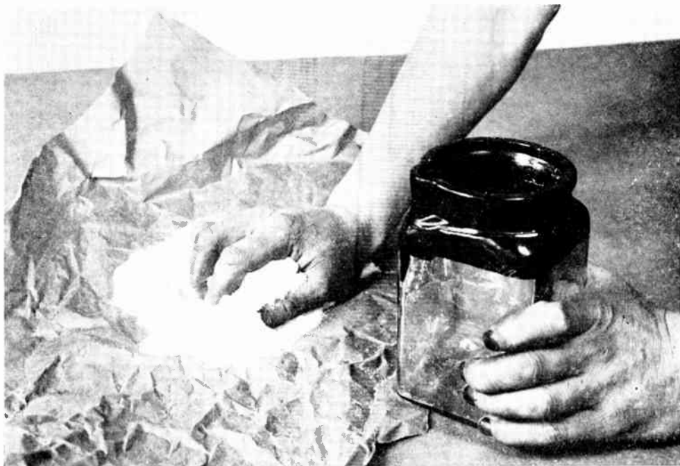
Fig. 1.—THE WRONG WAY OF MAKING UP SAL-AMMONIAC SOLUTION.
