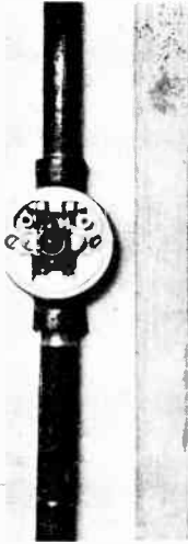
Fig. 10.—A SEMI-RECESSED "THROUGH" SWITCH BOX.
