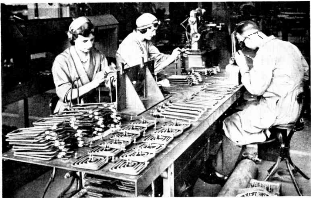
FITTING THE TERMINALS AND FERRULES TO THE TORRIBAR HEATING ELEMENTS.
