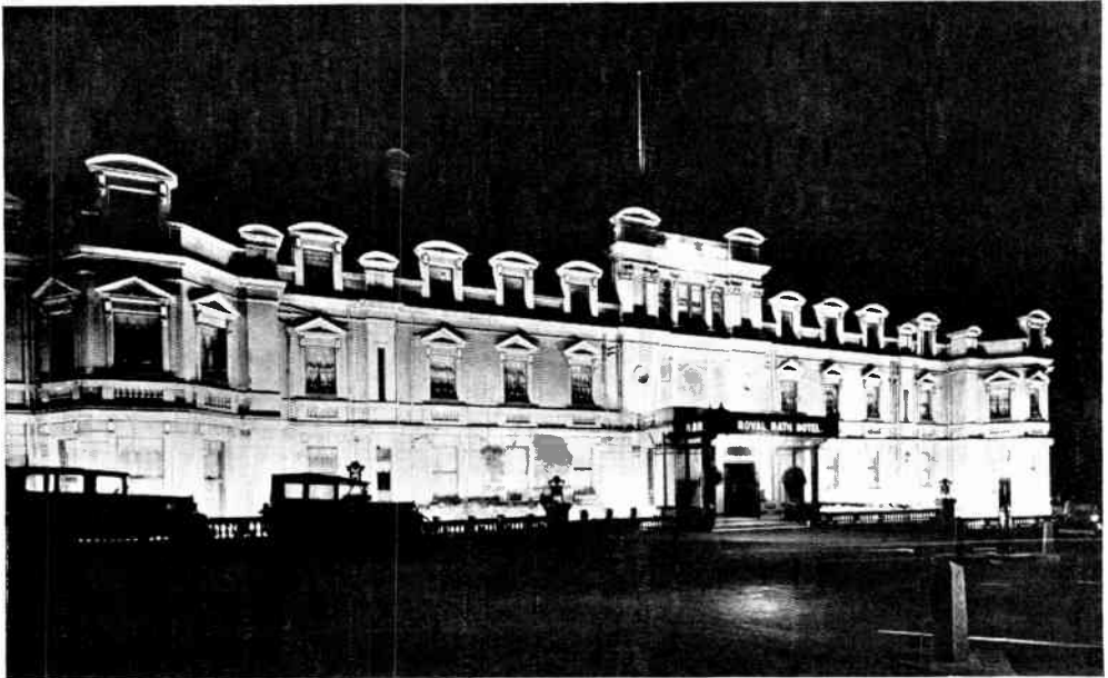
SHOWING THE USE OF MAZDA MERCRA LAMPS FOR FLOODLIGHTING THE ROYAL BATH HOTEL, BOURNEMOUTH.
