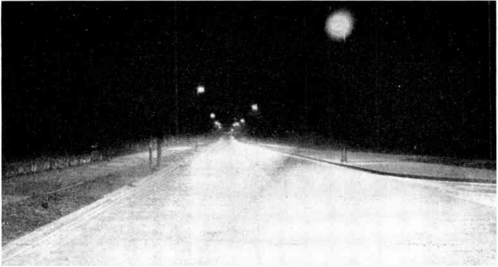
Fig. 1.—A SECTION OF THE WATFORD ROAD, WEMBLEY, MIDDLESEX, ILLUMINATED WITH OSIRA ELECTRIC DISCHARGE LAMPS.
