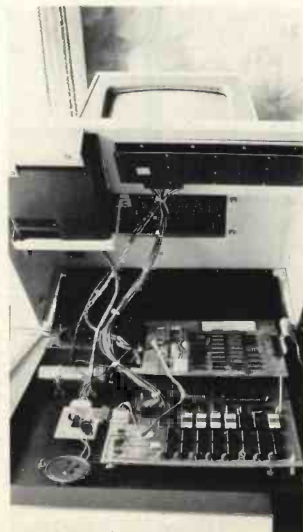
Inside the Pet. The 24K add-on memory is purpose-built. At left is the bleeper unit.
