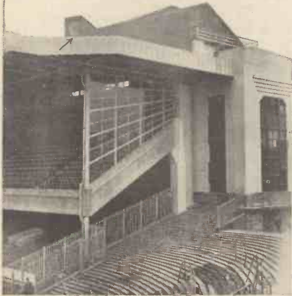
Marconiphone Photo] A portion of the great new stand at the Arsenal Football Club's ground at Highbury, showing one of the P.A. projectors (indicated by arrow).
