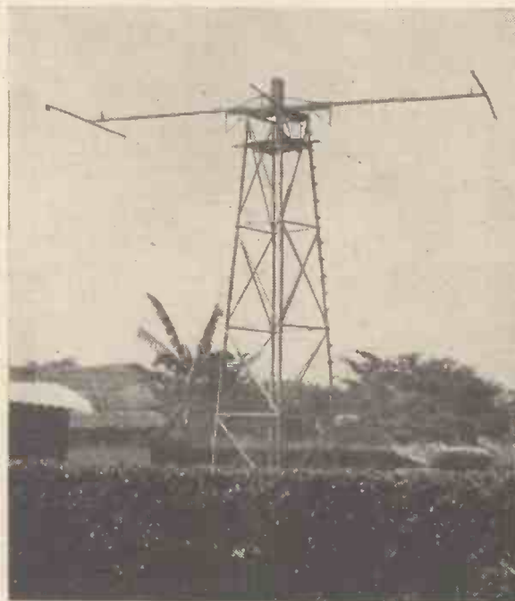
VU2DR, of Assam, India, attributes much of his success to his beam aerial, which he can rotate without moving from his seat at his operating bench. Quite a professional-looking affair, isn't it?
