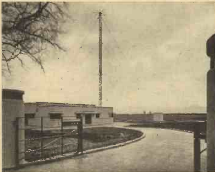
The station building and aerial mast at the new North Wales B.B.C. station at Penmon. The mast is 250 feet high and is surmounted by a red aircraft-warning light. Some interesting facts about the station are given on page 633.
