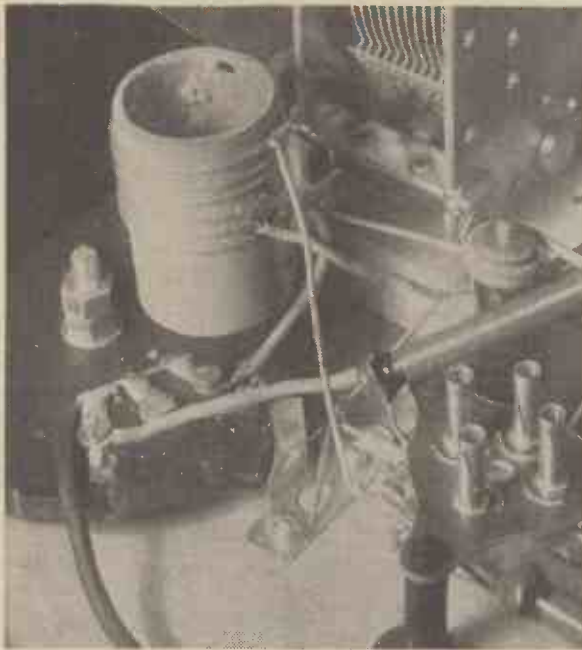
This photograph clearly depicts the method of coupling the aerial to the television coil. It will be seen that the wire from the aerial terminal to the B.C. coil is twisted round the terminal on the .0001-mfd. fixed condenser.
