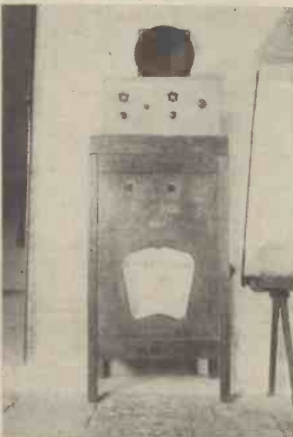
Good workmanship in the Far East. A photograph received from S. C. G. (Gloucester), of a set used by him in Singapore. It has the W.L.S. one-valver as a basis, but now boasts four valves.
