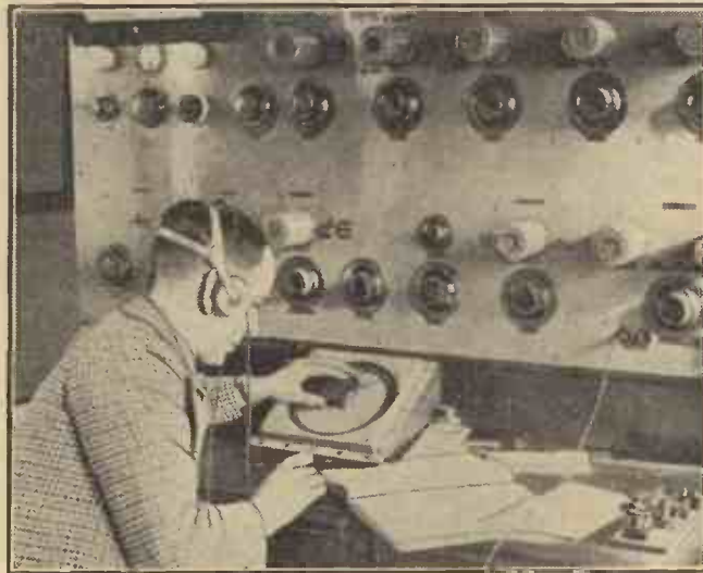
The new direction-finding receiver at Fulham Air Station, Norfolk. The apparatus is used in conjunction with that at Croydon and Lympne, and provides air pilots with a means of readily ascertaining their position.
