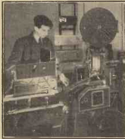
A 180-line Baird scanner for use in the transmission of films by television.
