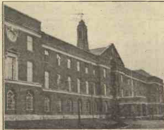
A view of the magnificent new G.P.O. Research Laboratory at Dollis Hill, which was recently officially opened.
