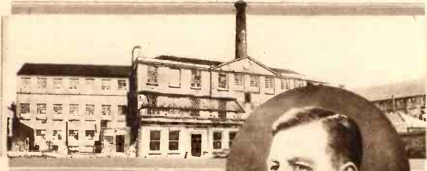
A portion of the fine new factory which was built last year to keep pace with the demand for W.B. products.
