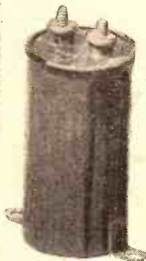
The Dubilier non-inductive fixed condenser which is an indispensable item in many band-pass sets.
