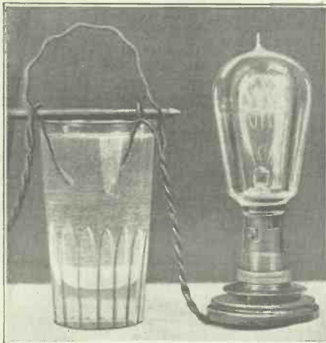
How the water test is carried out.
