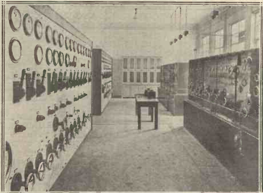
Here are the two 20-kw. short-wave transmitters at the Nauen station in Germany. Nauen's call-sign is A G C, and it operates on 17.20 metres.
