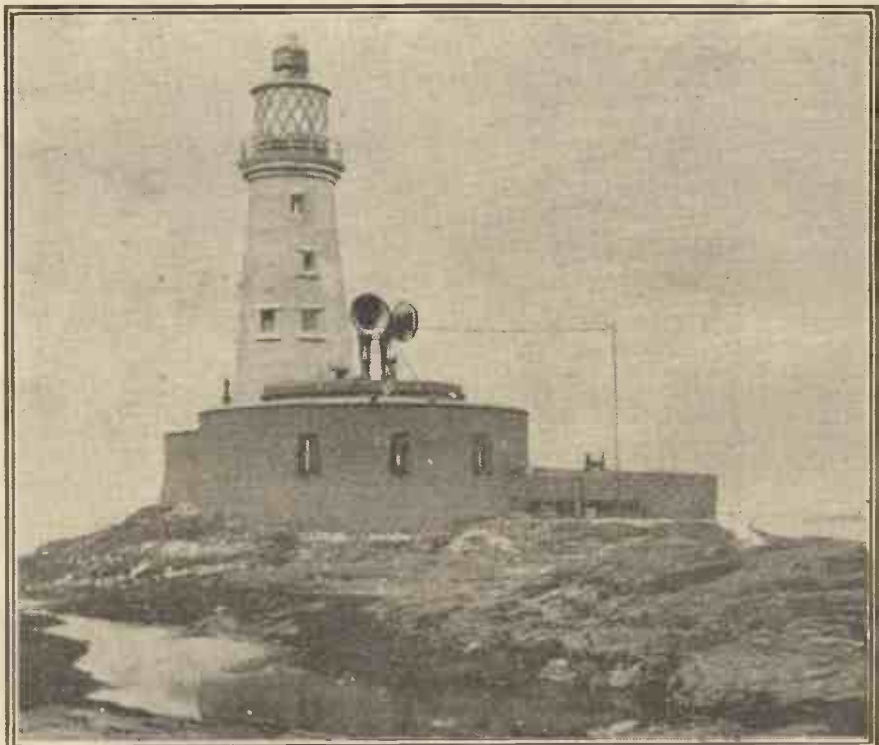
The Longstone Lighthouse, where Grace Darling lived, on the outer Farnes Islands, in the North Sea. The three light-keepers have recently erected an aerial to enable them to listen to the outside world.
