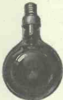
Fig. 3.—An American photo-electric cell of the vacuum type.
