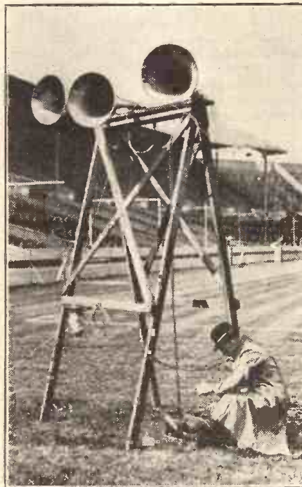
An engineer installing loud speakers and a microphone at Wembley preliminary to the broadcasting of a big sporting event (Marconiphone).
