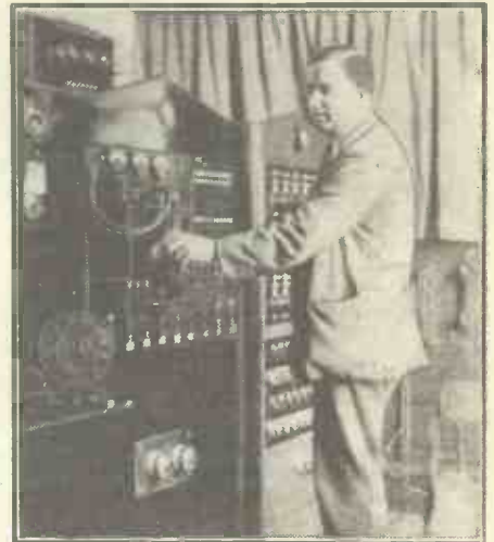
Mr. F. Stevens, in the Control Room.
