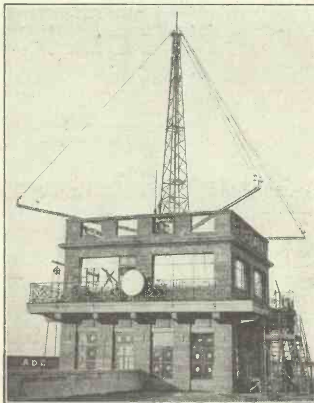
It is claimed that the new aerodrome at Croydon will be the best-equipped terminal air station in the world. In the mystery tower three people will be on duty day and night, and will have control over air expresses flying hundreds of miles distant. Above the control tower is the mast of a perfected wireless installation which will enable those in it to tell pilots who are in flight where they are, and guide them to Croydon in any weather.
