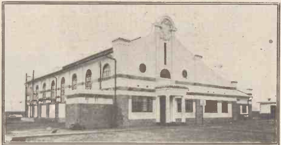
The Power House of the Klipheuevel Transmitting Beam Station, which is situated 30 miles N.E. of Cape Town.
