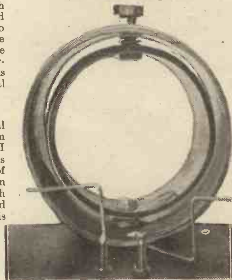
Fig. 2. Both ends of the rotor winding should be soldered to the shaft of the spindle.
