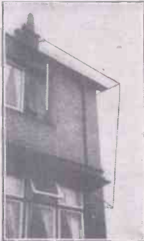
Making the best of cramped quarters. The aerial cannot come direct to the set and is kept away from the building by insulated supports.
