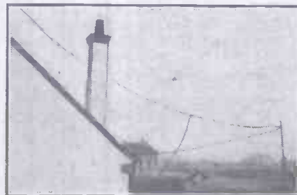
Two aerials on one mast are to be avoided if DX results are desired.
