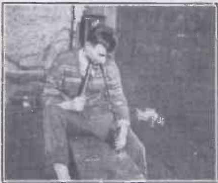
Installing the aerial upon the roof of Mr. Ramsay MacDonald's house at Hampstead.
