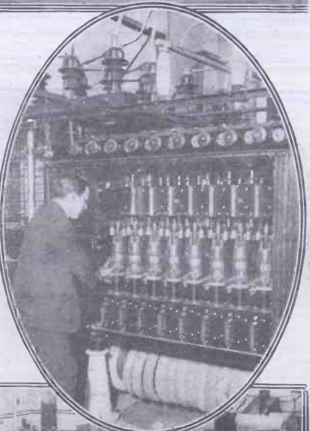
(Left). Setting one of the controls on the D.C. switch cubicles at Rugby. (Right). This photograph shows one of the valve power units with its bank of water-cooled valves. These units are protected by sliding iron gates, one of which can be seen on the right of the picture. Note the large insulating pillar supporting the panel.
