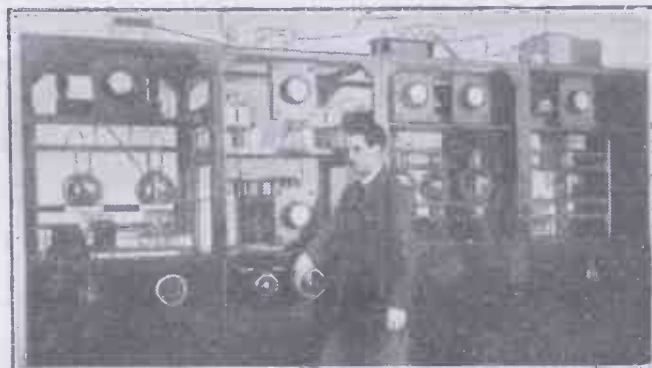
A section of the transmitting apparatus at the Riga broadcasting station.
