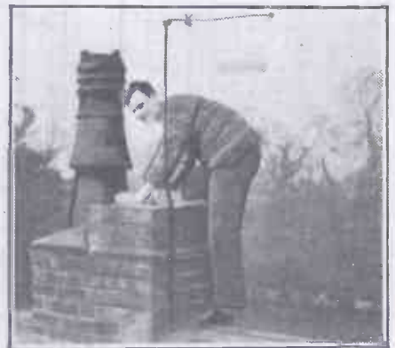
This is not Father Christmas, but another view taken upon the ex-Premier's roof. Readers will notice that he chose Winsulators!
