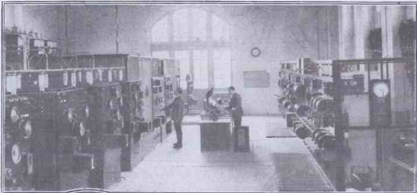
A corner of the valve room, showing the power units, exciter panels and control table.
