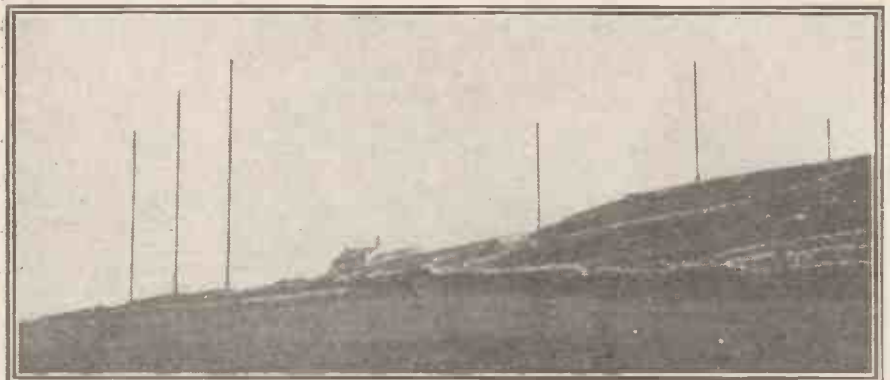
The masts of the Marconi Co.'s giant station at Carnarvon, Wales.
