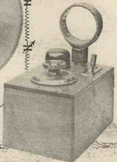
The Dubilier Buzzer Wave-meter. Price £5:5:0 } For wave-lengths from 100 to 3,000 metres.
