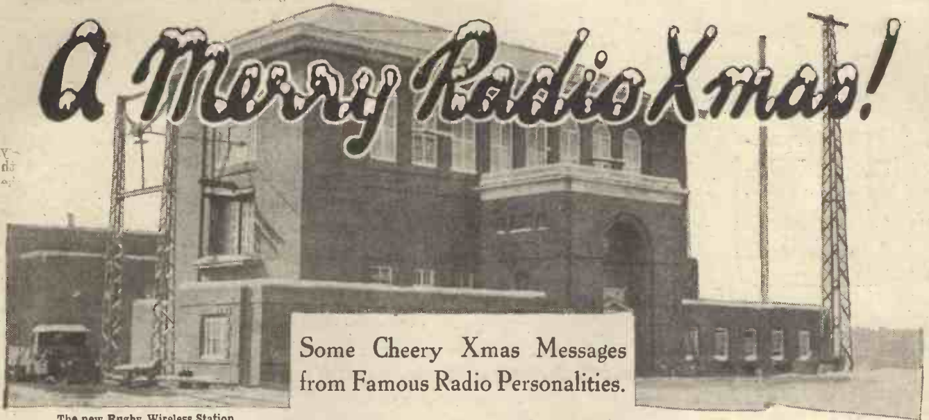
The new Rugby Wireless Station.
