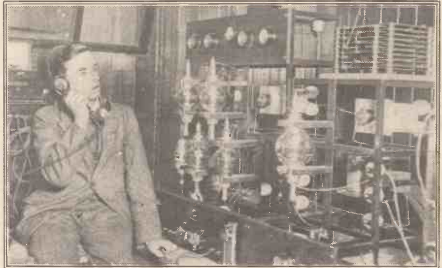
Mr. Beveridge, engineer-in-charge of the Edinburgh wireless station, and part of the transmitting gear.
