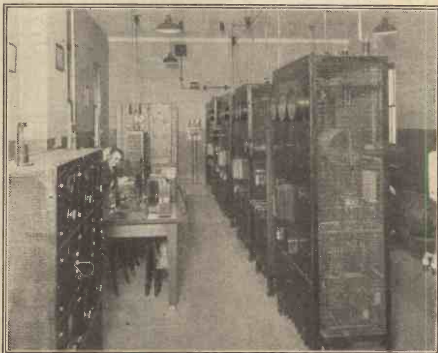
The transmitting-room of W J Z, the well-known broadcasting station at New York. This station transmits on 455 metres with a power of 500 watts.
