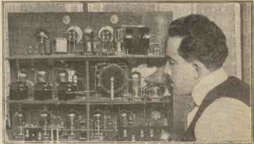
A twelve-valve super-heterodyne receiver as constructed by an American amateur.
