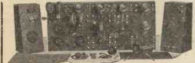
Showing the Assembly of a Five-Valve Receiving Set.
