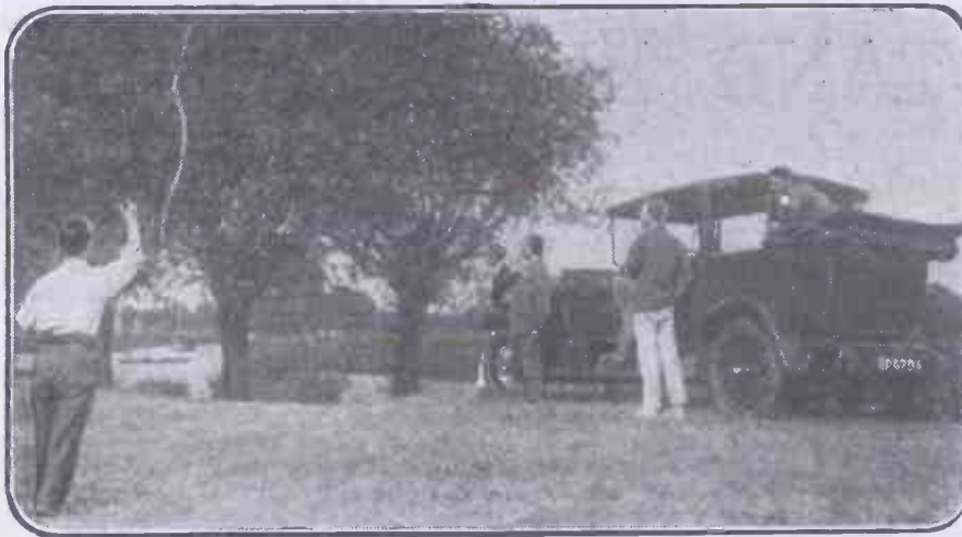
Hoisting the aerial by throwing the line with a bottle attached into a tree.
