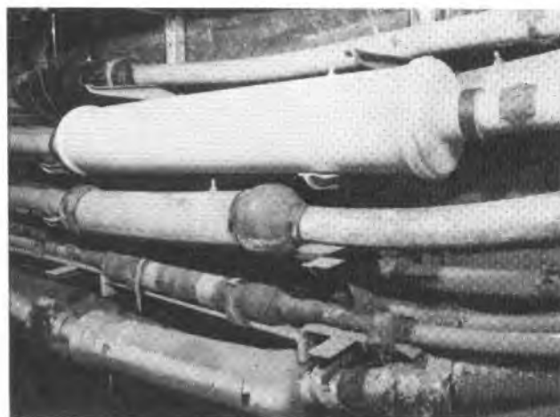
FIG. 2—The renewed closure showing the single-cable-entry end
