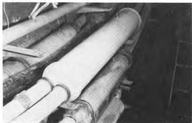
FIG. 3—The renewed closure showing the twin-cable-entry end
