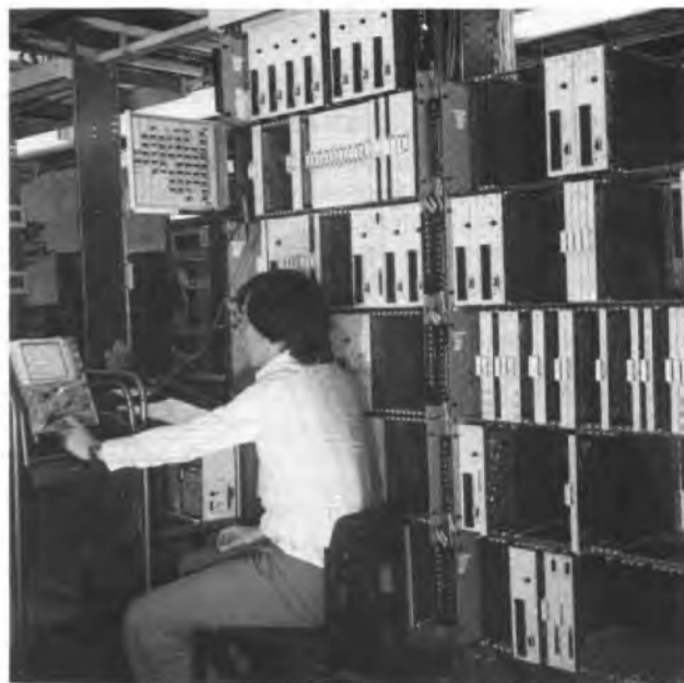
FIG. 3—A small processor utility being commissioned
