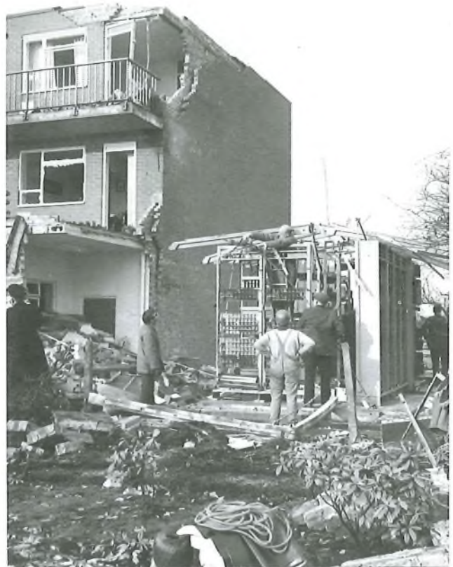
FIG. 1—Madeley exchange after gas explosion
