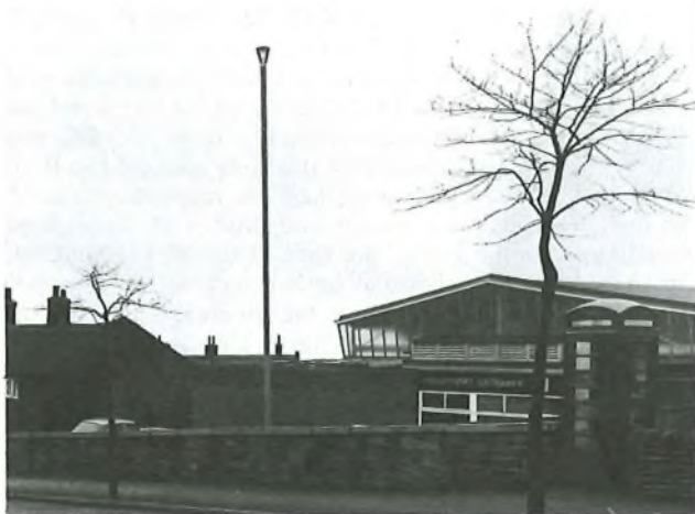
FIG. 4—Vent pipe at exchange manhole
