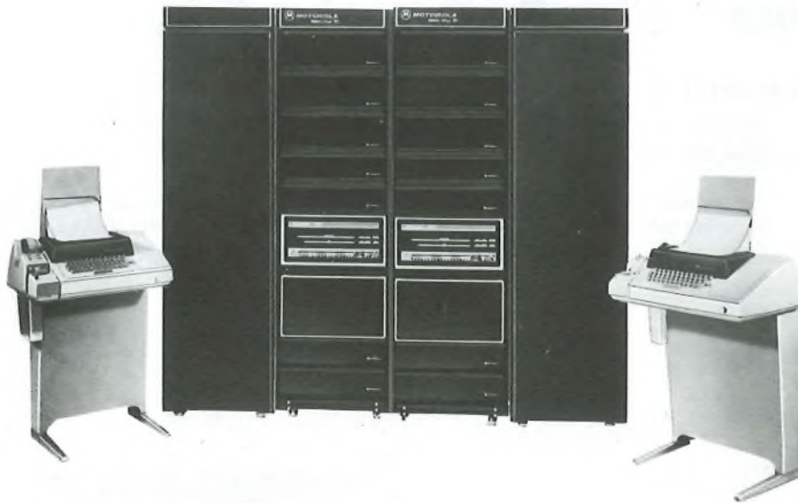
FIG. 2—The paging control equipment
