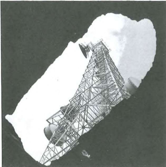
The tower viewed through the damaged roof of the radio station
