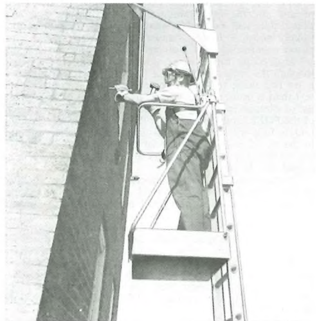
FIG. 5—The ESSVE Combined Ladder and Platform on field trial
