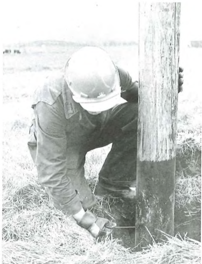
FIG. 2—Pole testing: inspection around the soil line
