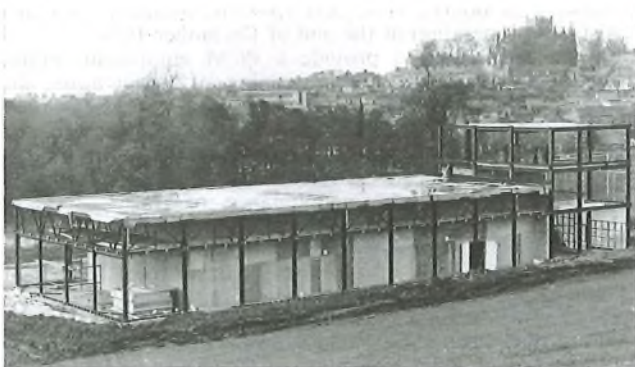
Wooden cocoon within the steel framework, 1 month before equipment installation commenced
