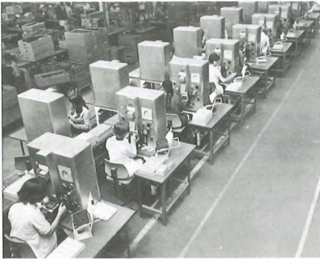
FIG. 8—Hot-press printing flowline
