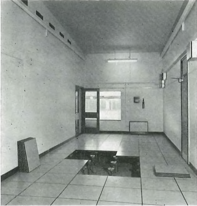
FIG. 3—Raised floor system used for the prototype M building showing adjustable metal stools with cruciform plastic tops designed to prevent individual covers slipping when the floor is open
