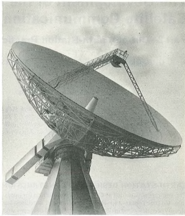
FIG. 3—Aerial at Hong Kong, built in 1969. The high-level azimuth track at the top of the concrete tower can be seen clearly.
