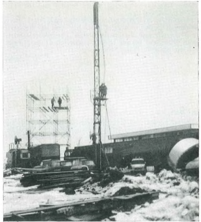
Erection of the scaffold platform with temporary BBC aerial in the foreground
