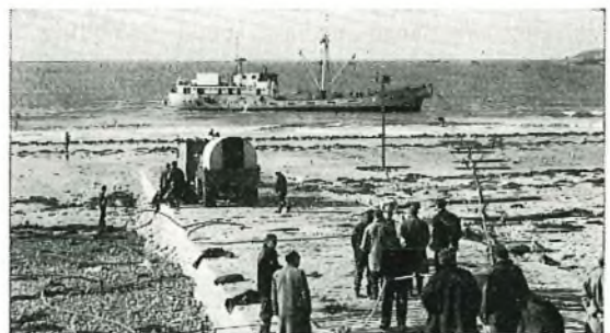
The Jersey end of the cable being taken ashore from the Cables ship Poolster.
