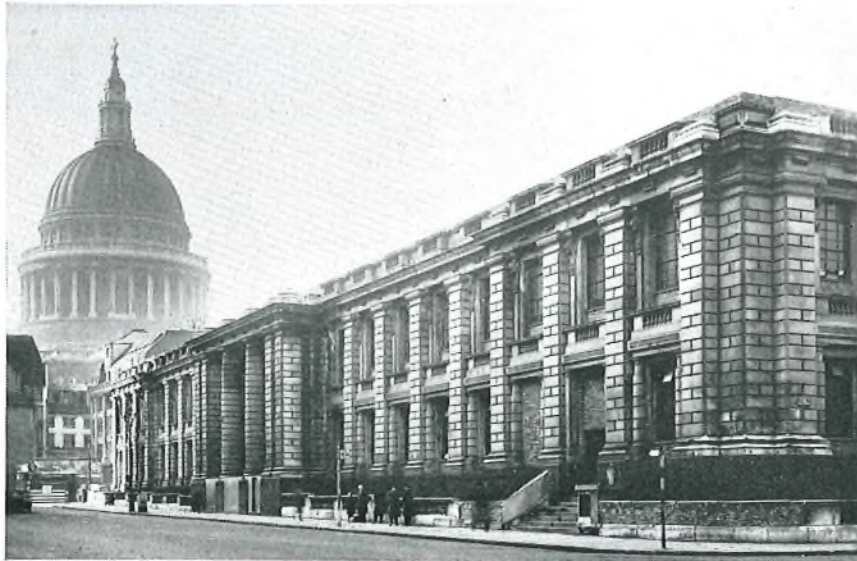
FIG. 3—THE C.T.O. AFTER REBUILDING
