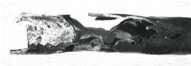
FIG. 7—POLYTHENE-SHEATHED CARRIER-FREQUENCY CABLE ATTACKED BY TERMITES ( MACROTERMES BELlicosus )
