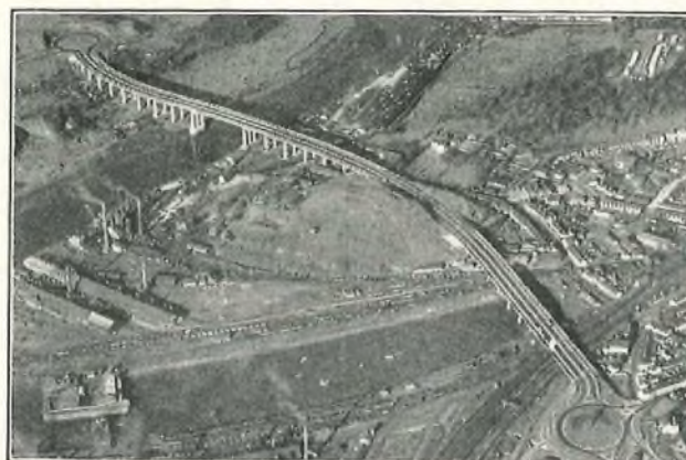
FIG. 2.—AN AERIAL PHOTOGRAPH OF THE NEATH RIVER BRIDGE AND ITS APPROACHES. BRITON FERRY IS ON THE RIGHT OF THE PICTURE.
