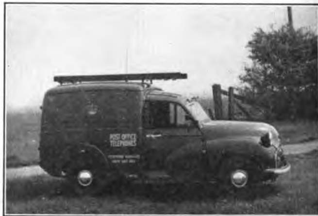
VEHICLE, SHOWING POSITION OF AERIAL.
