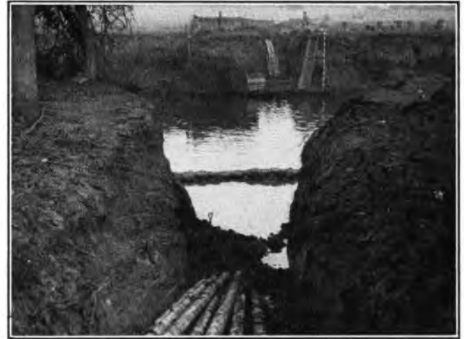
PIPES LAID IN CHANNEL ACROSS AVON.
