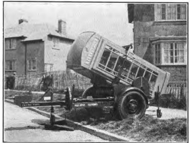
FIG. 5.—PLACING A KIOSK ON SITE.
