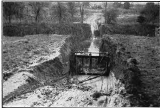
DREDGING THE CHANNEL ACROSS RIVER AVON.
