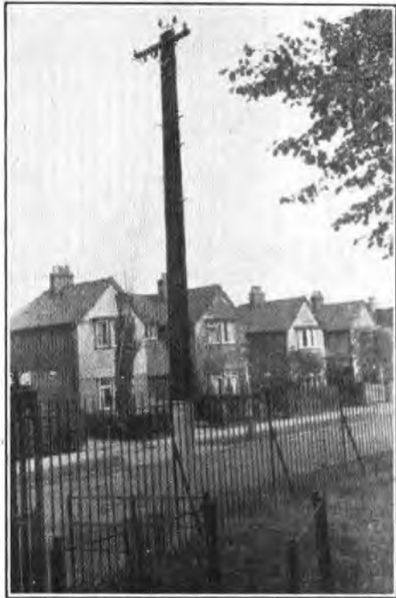
"HALVED" POLE ERECTED.
