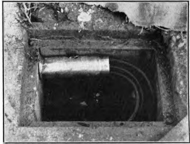
FIG. 5.—SEALED JOINT PLACED IN JOINT-BOX.
