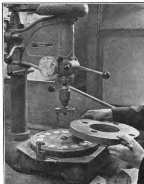
FIG. 1.—DRILL-PRESS LAP.
