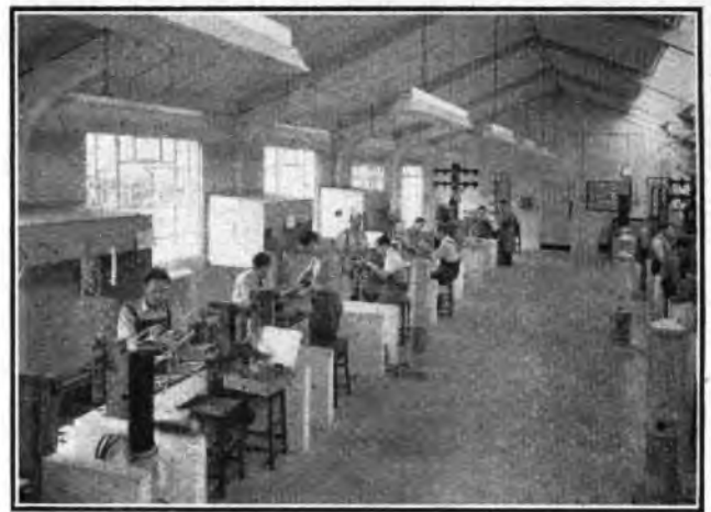
FIG. 3.—UNDERGROUND JOINTING ROOM.
