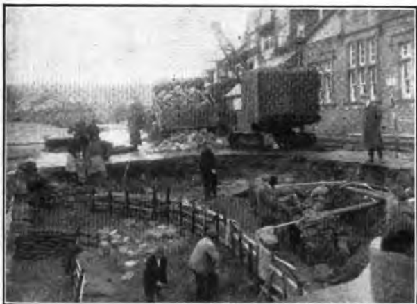
REPAIRS IN PROGRESS AFTER DEMOLITION OF JOINT BOX.
