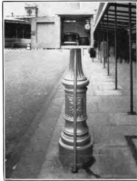
FIG. 8.—TELEPHONE ON LAMP-POST FOR CAR-CALL SERVICE.
