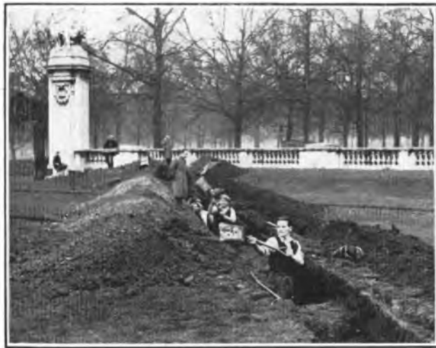
FIG. 2.—EXCAVATING FOR DUCT ROUTE NEAR CANADA GATE.
