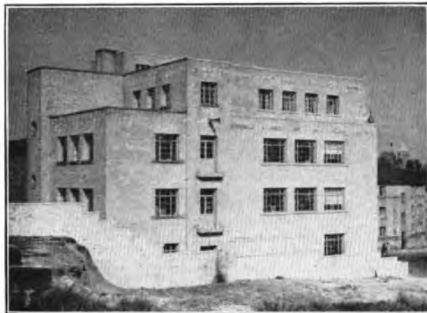
GREENOCK AUTO EXCHANGE BUILDING.
