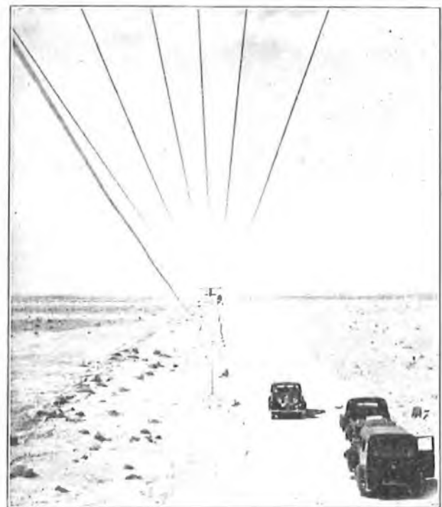
FIG. 3.—VIEW OF A SECTION OF THE LINE.
