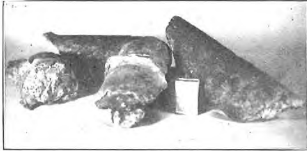
FUNGUS FORMATION REMOVED FROM DUCT.
