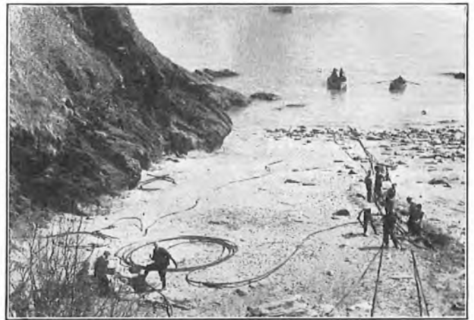
TESTING ONE OF THE SHORE ENDS.
