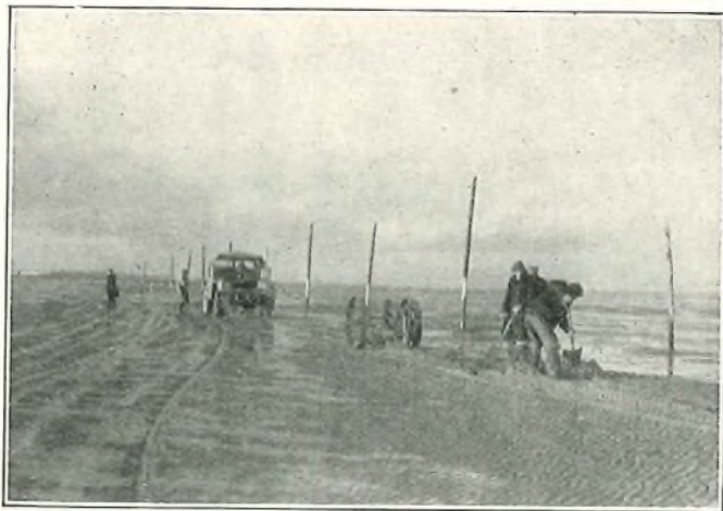
CABLE LAYING IN PROGRESS ON THE "SEA" SECTION.
